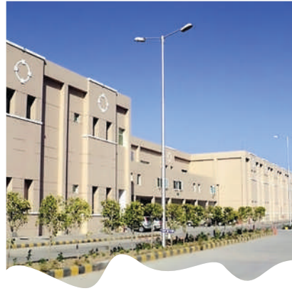
Patanjali Industrial Park
